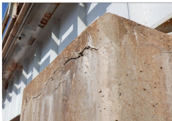
Figure 6. Concrete Failure on SH-99 over Cimarron River Bridge
