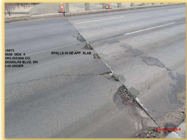
Figure 3: Douglas Boulevard Bridge Deck
