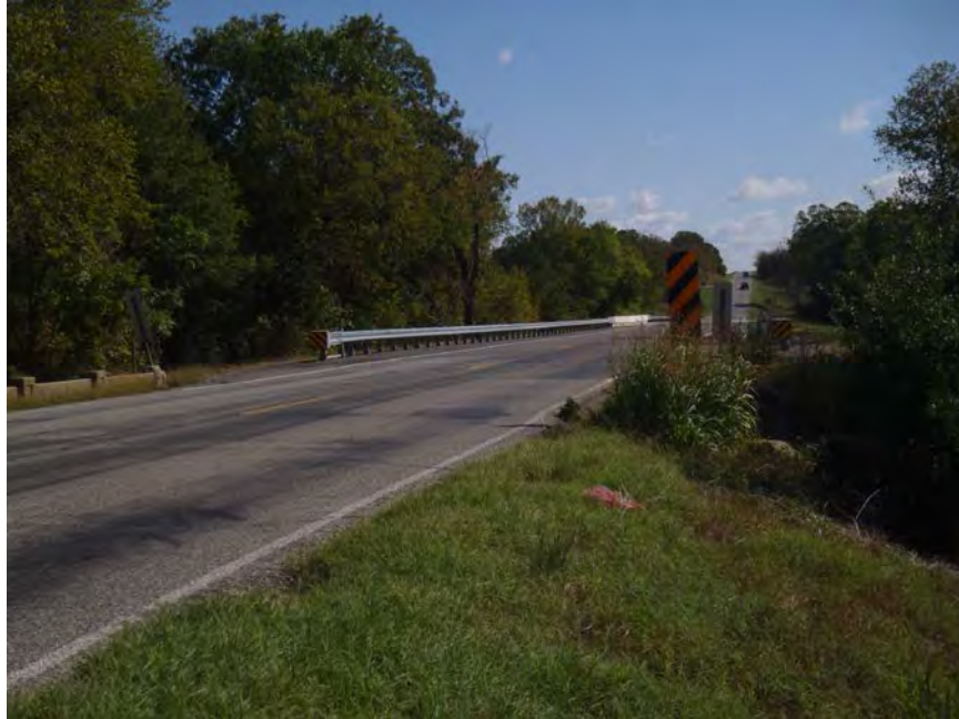
NBI # 06295 in foreground and recently completed Watson Creek Bridge
