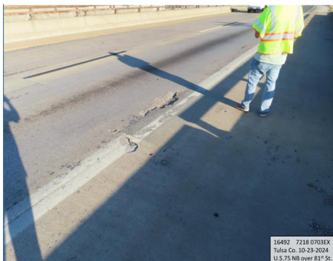
Figure 8: NBI#16492, Spalling of Bridge Deck
