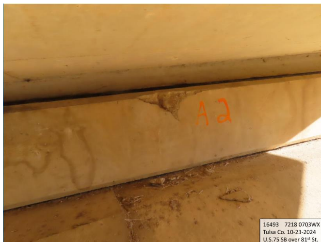
Figure 10: NBI#16493, Spalling of Support Beam
