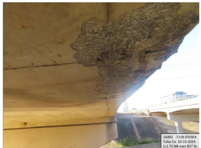
Figure 9: NBI#16492, Spalling of the Bridge Soffit
