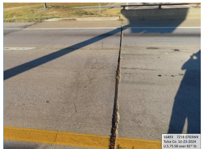
Figure 11: NBI# 16493 Cracks on Expansion Joint
