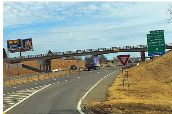
Photo 8: View of Engle St. bridge from I-40 facing eastward.
