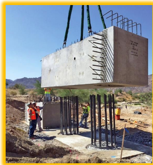
Figure 20 – Construction with Pre-Cast Abutment
