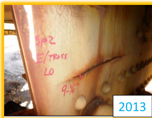
Figure 4 – Worsening Cracks and Corrosion in gusset plates
