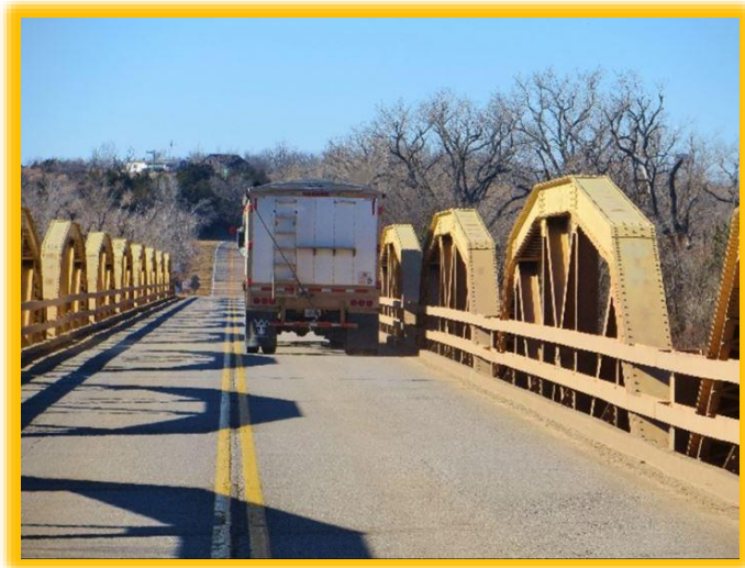
Figure 15 – Heavy Truck Traffic on the Bridge
