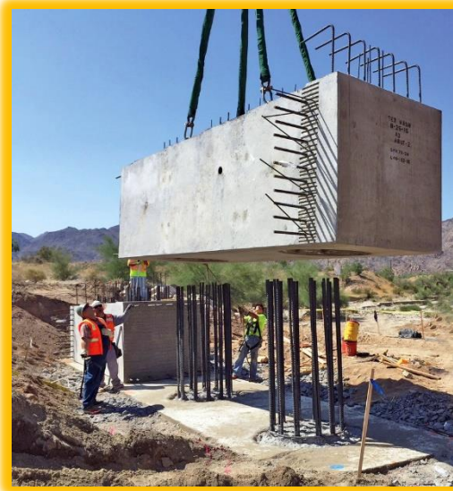
Figure 13 – Construction with Pre-Cast Abutment
