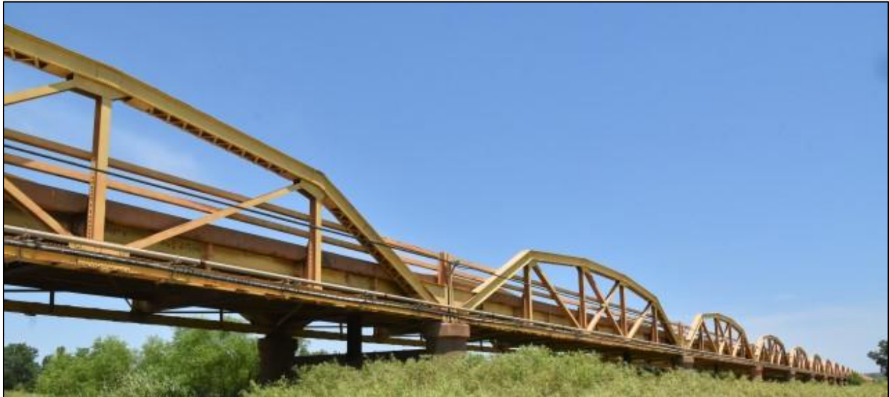
Figure 2 – Bridgeport Bridge ( historicbridges.org )
